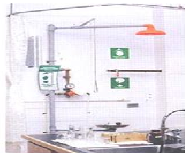
Figure 2 Lab eyewash stations and emergency showers can rinse off chemicals quickly.
