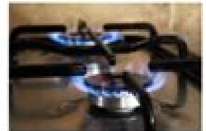
Natural Gas Heating
