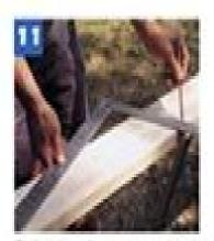
To find the rafter cutting angle, align the 5- and 12-in, marks on the framing square's legs with the edge of the rafter stock.
