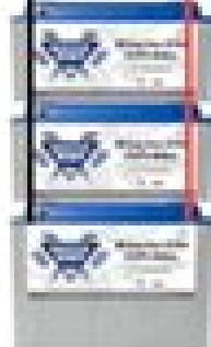
3x Battleborn Lithium Batteries in Parallel (300Ah)
