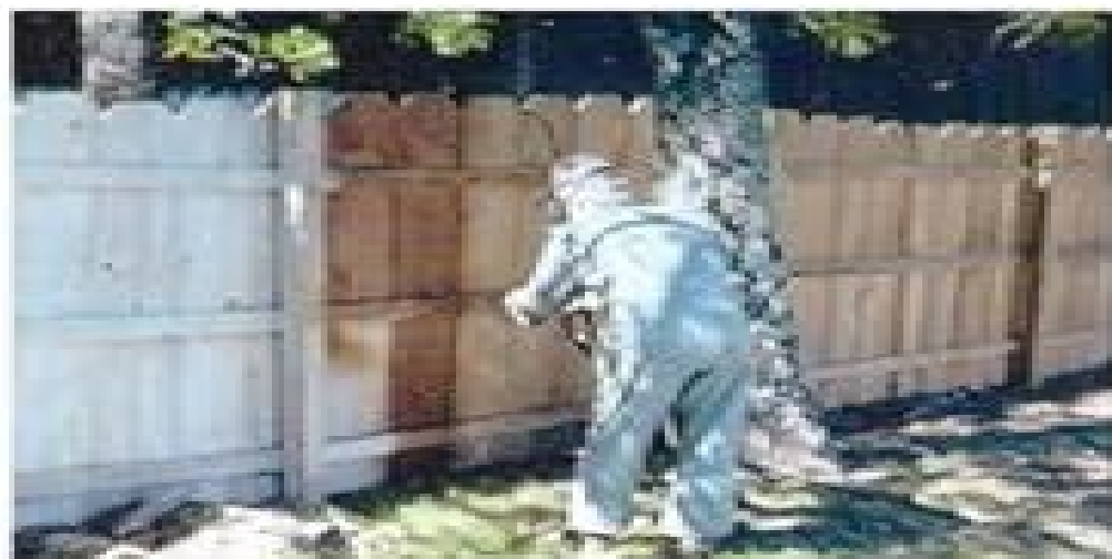
Applying FMP 220 Series Coolstone Moisture to a cleaned, weathered cedar fence.
