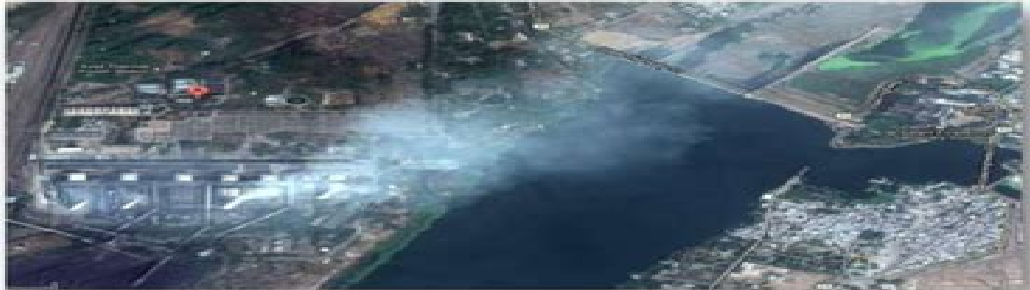
BIRD VIEW OF KOTA THERMAL POWER PLANT, RAJASTHAN, INDIA
